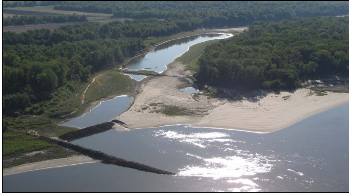
Looking downstream at the entrance to Salt Lake Chute RM 139.2
