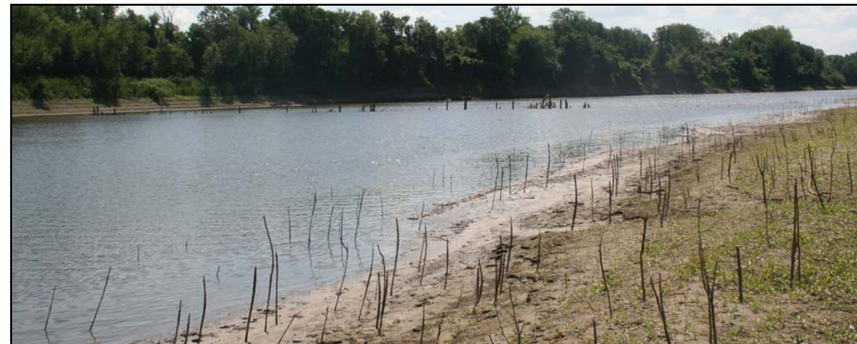
Looking upstream in Salt Lake Chute at Pile Dike 138.45L
