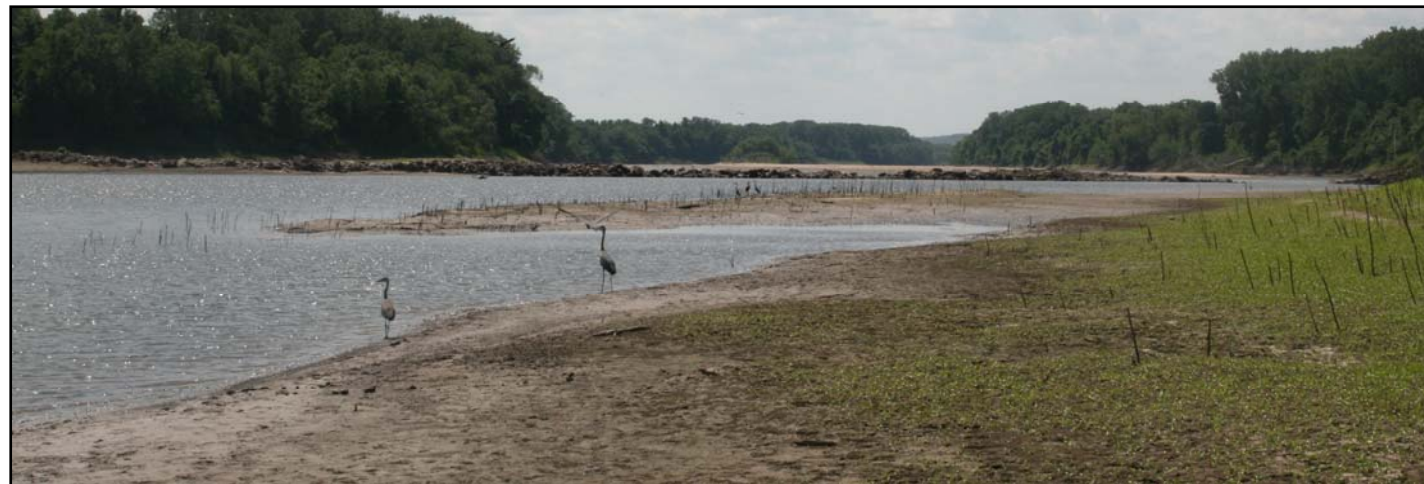
Looking upstream in Salt Lake Chute at Dike 138.1L
